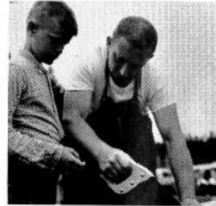
Shop activities include building log cabin with Ted's assistance . . .
